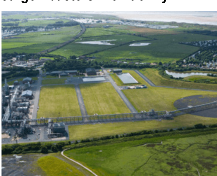
Image of Point of Ayr Terminal
